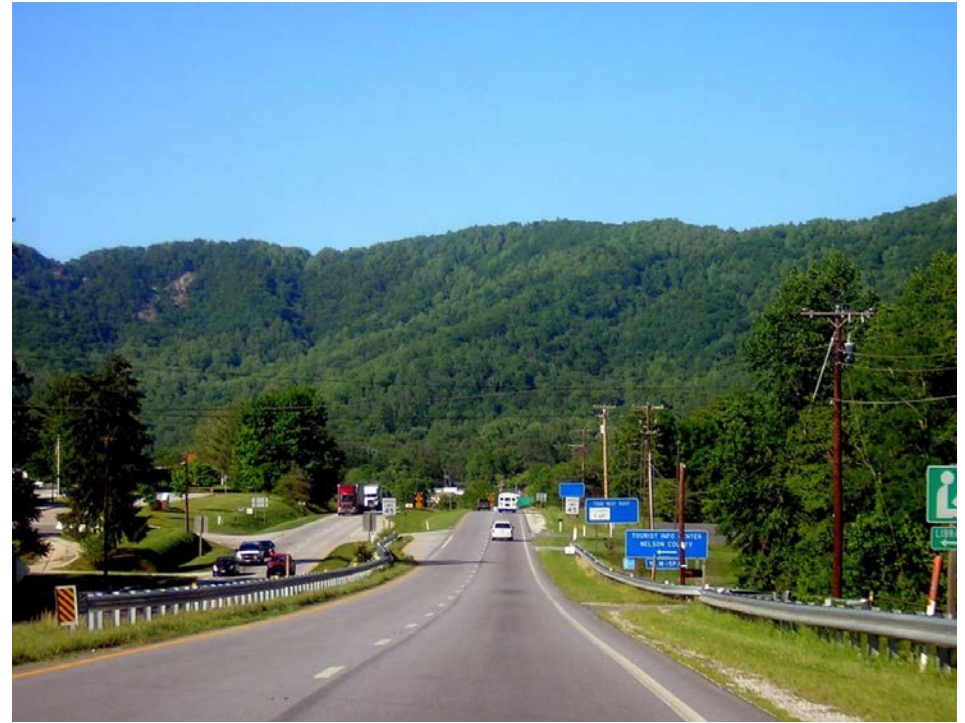
View of U.S. 29 in Lovington. Image courtesy panorramio.com
