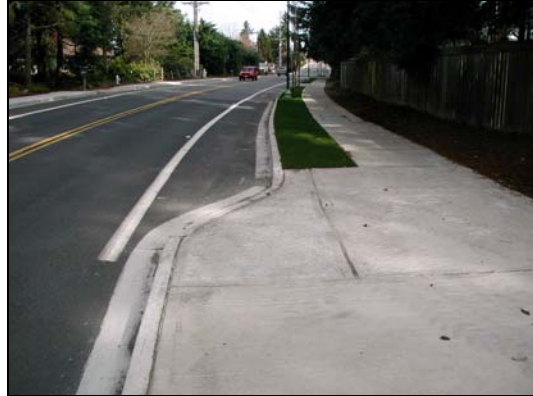
Bike lanes approaching roundabouts can have their own ramp onto the sidewalk, though most experienced riders will prefer to merge with the slow-moving traffic. (Dan Burden)
