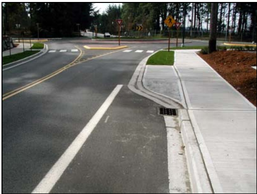
Bike lanes approaching roundabouts can have their own ramp onto the sidewalk, though most experienced riders will prefer to merge with the slow-moving traffic. (Dan Burden)
