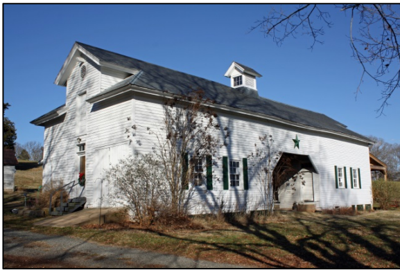
Figure 31- The barn at Garnkirk (062-5135-0055)
