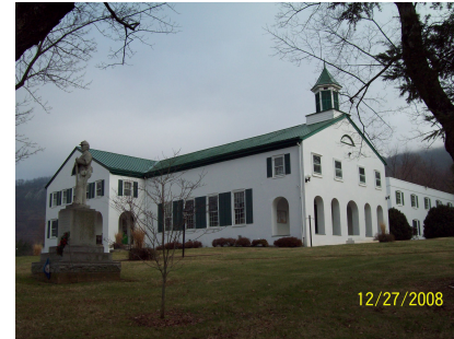
Source: Wikipedia, "Nelson County Courthouse," http://en.wikipedia.org/wiki/Nelson_County_Courthouse
